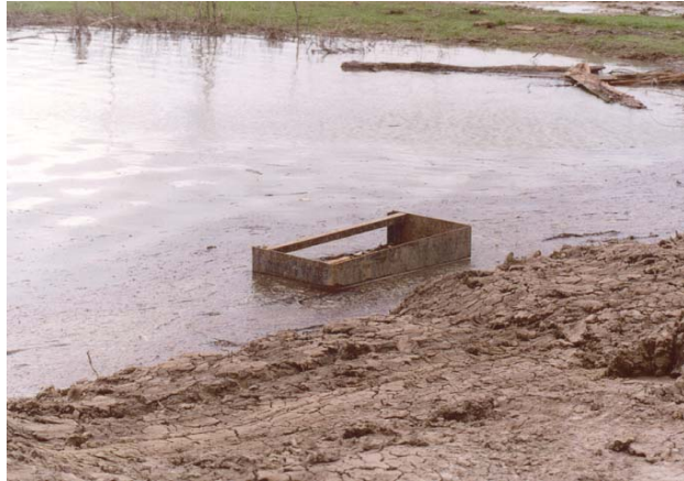
WCS stopping sediment
